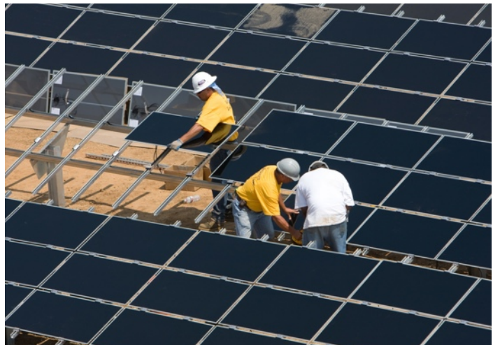
Workers from renewable energy company enXco install panels on a 1-megawatt solar array on a turkey farm near Wilton, CA. The array provides power to subscribers of the Sacramento Municipal Utility District's SolarShares program. Photo courtesy of SMUD.
